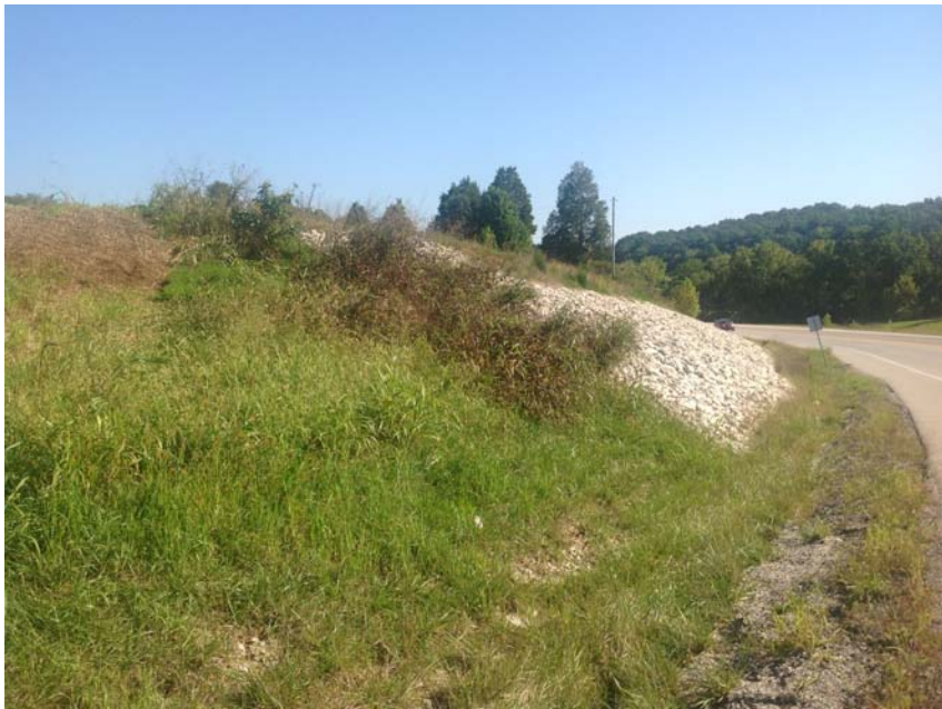
Landslide repair on relatively flat slope underlain by poor shales on KY 89 near Clay City.
