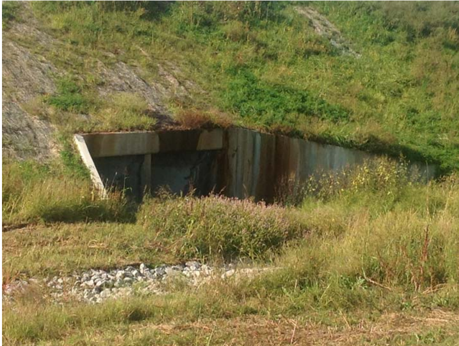
Box Culvert under Mountain Parkway Ramp near Kiddville showing staining due to Acidic runoff from New Albany Shale Backfill.
