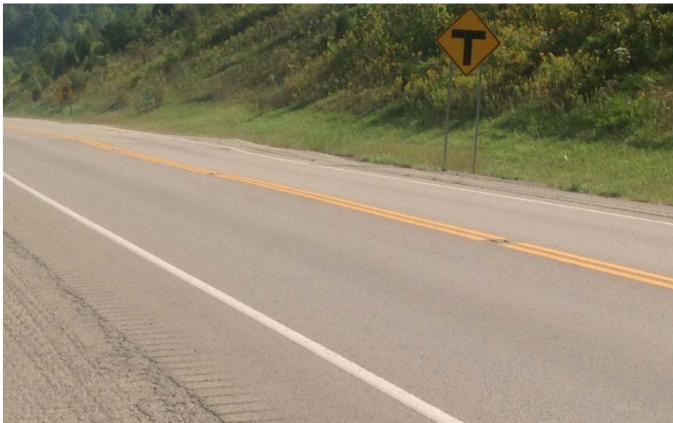
Irregular (wavy) Pavement due to swelling shales on KY 499
